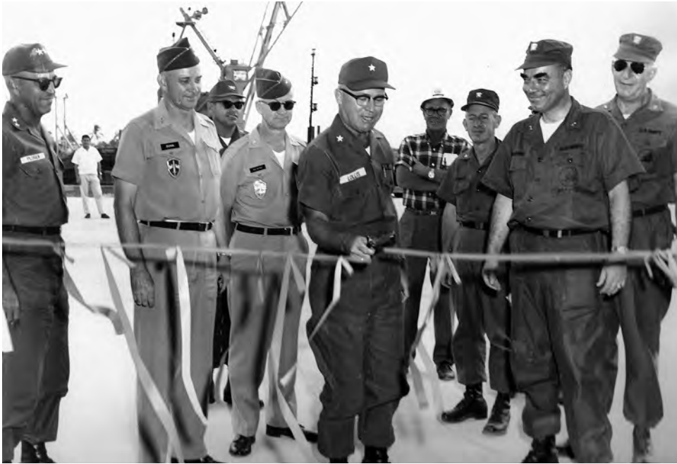
A ribbon-cutting ceremony marked the opening of the Newport deep-draft port facility in Saigon when Brig. Gen. Shelton E. Lollis, commanding general of the 1st Logistical Command, officiated by cutting the ribbon as (left to right) Generals Ploger, Dunn, and Raymond and Admirals Husband and Seuffer observe.
